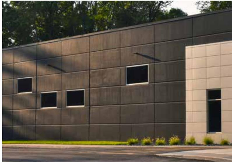
▲ Certain angles of sunlight can expose panel variations even as small as 1 mm—about the thickness of a dime. This does not affect the functionality of your panel.
